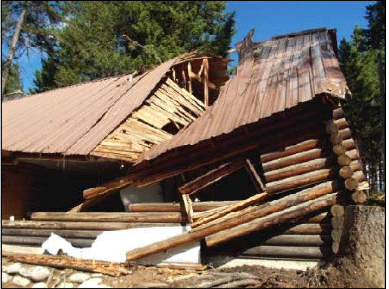
**Figure 8: Close up view of damage to east half of Mess Hall.**
